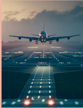
Airfield Lighting Cables
